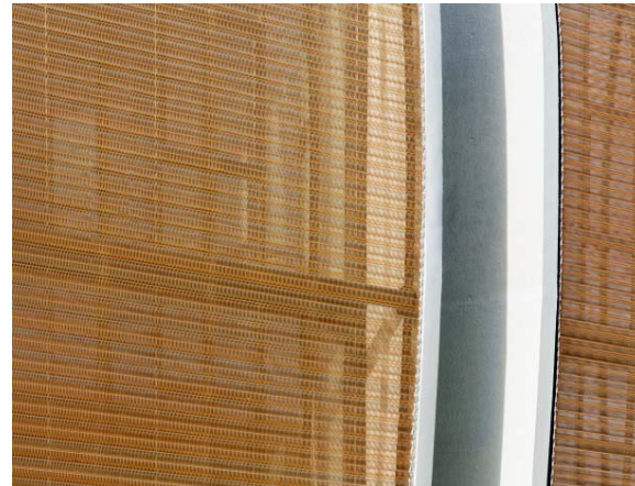
Picture 5: Suspended façade elements made of gold-colored aluminum mesh from GKD.
