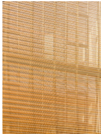
Picture 3+4: The semi-transparent metal mesh from GKD performs the function of a protective membrane between the outside world and the internal life of the school.
