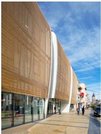
Picture 3+4: The semi-transparent metal mesh from GKD performs the function of a protective membrane between the outside world and the internal life of the school.
