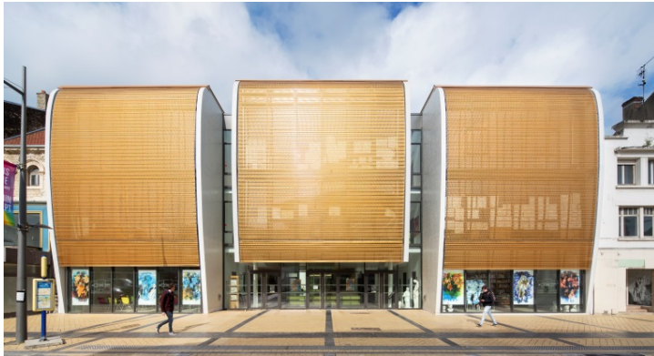
Picture 1: Curved solar protection façade in three pieces made of golden Escale metal mesh from GKD at the Ecole d'Art de Calais.
